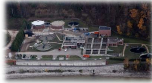
Wastewater Treatment Plant after addition of tank domes
