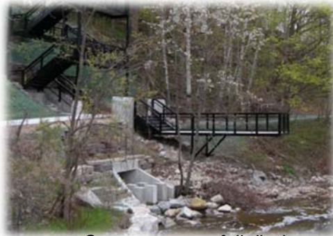
Storm sewer outfall dissipater
