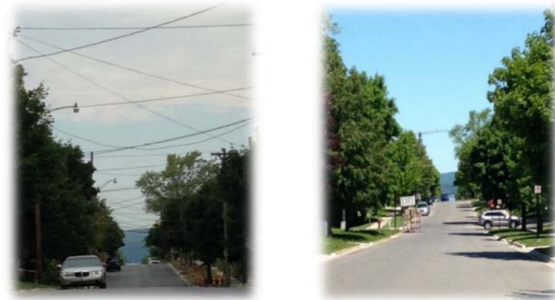
Emmet Street before and after electric lines buried
